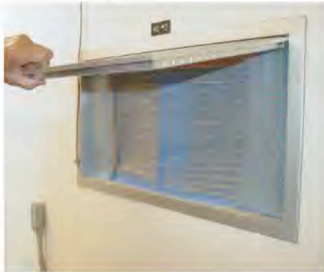
Fig. 3: Summer is a good time to check and replace dirty air conditioner filters.
